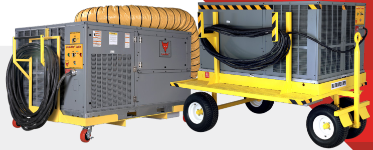
MOBILE CONFIGURATION (Shown in Trolley and Trailer Mounted Configuration)
